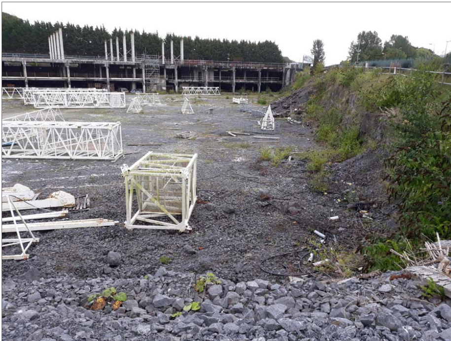
Plate No. 11.4 South-west corner of subject site, from N
