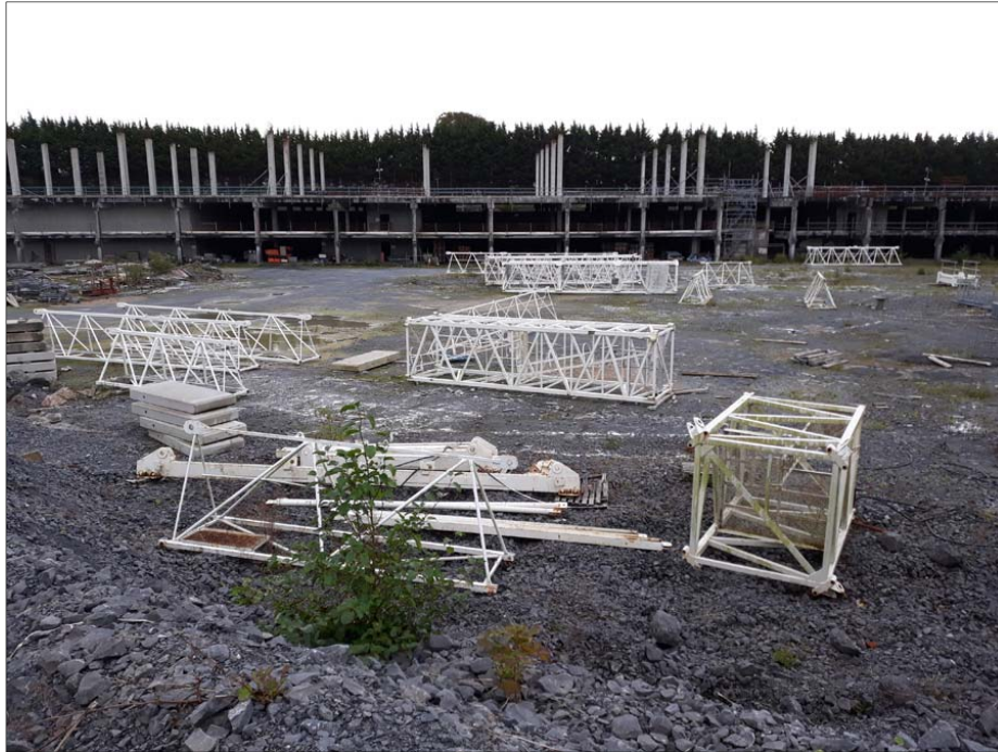
Plate No. 11.5 Partially constructed car park at S side of subject site, from N
